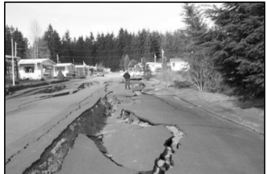
Image of damage from the 2001 Nisqually earthquake near Seattle
