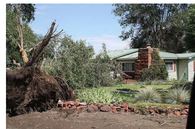
A tree came crashing down in front of a residence during the Aug. 25, 2013 storm.
