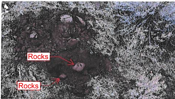
Picture 19 – Test hole, Loamy Sand with cobbles at 6 inches.
